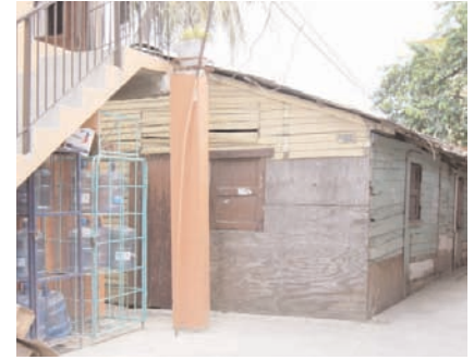
Original Wooden House
